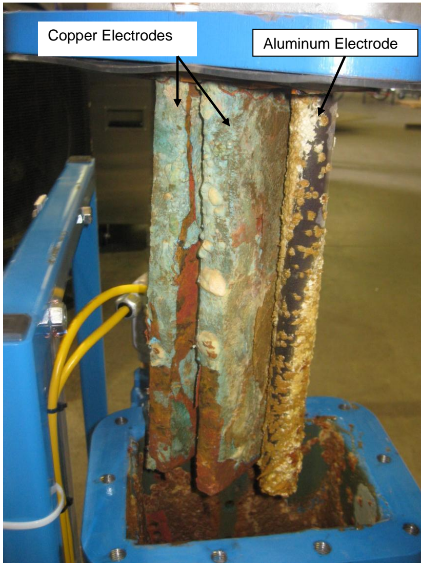
Figure 23 Lid of ion generator removed exposing the scale coated copper and aluminum electrodes
